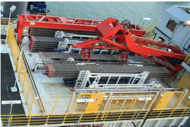
Automated pipe storage area with pipe feeder.
